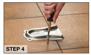
Position each caster positioning chock into their final location and secure with screws.
