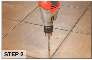
Using a 3/8" bit, drill 3/4" through each point. Place an anchor in each hole. Ensure they are flush.
